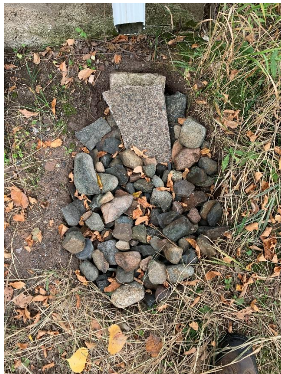
Settling Pit Completed
